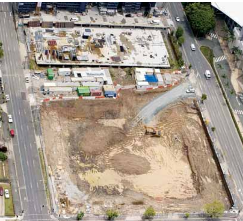
ABOVE: The SW1 site works, South Brisbane.
